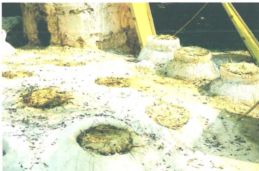
**Photo.15. Pressing the dried straw down with Lime in earthen pots**
